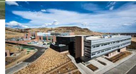
Energy Systems Integration Facility Golden, Colorado
